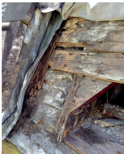
Rotten sarking caused by a failing skew abutment
