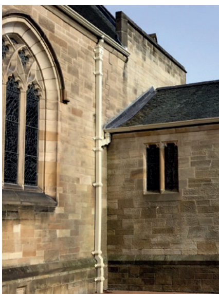
Rainwater goods replaced with larger cast iron sections and a wide watertight detail to cope with increased rainwater
