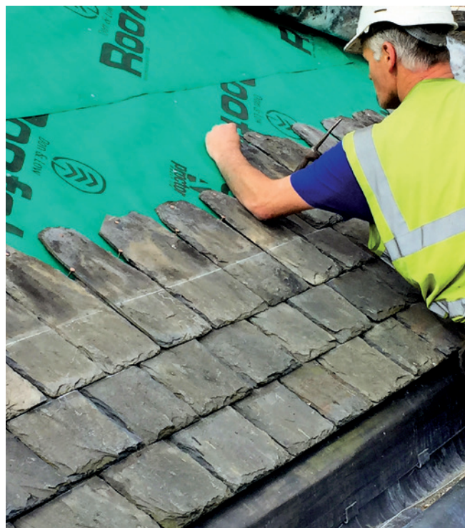
A roofer cheek nailing slates on an exposed roof
