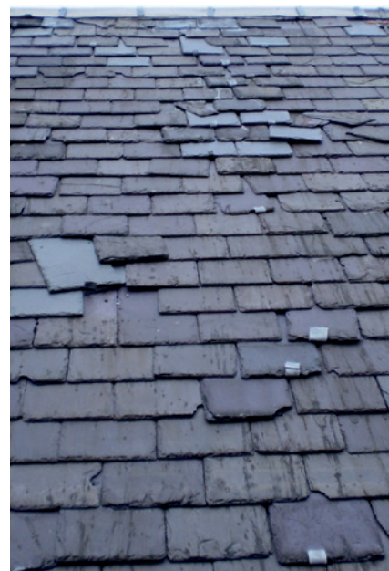
A wind-damaged slate roof with tingles and a variety of other poor repairs
