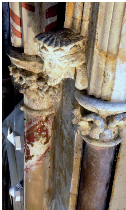
Salt crystallisation damage at a high level caused by warm, moist air condensing on cold fabric
