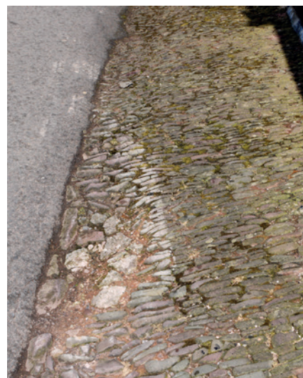
Another inappropriate repair using mismatched stones
