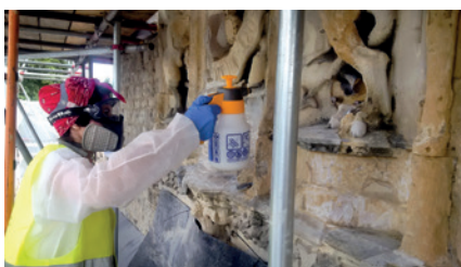
Nanolime was applied with a pressurised garden spray and the area was covered in cling-film between applications to delay evaporation of the ethanol and promote maximum penetration.
