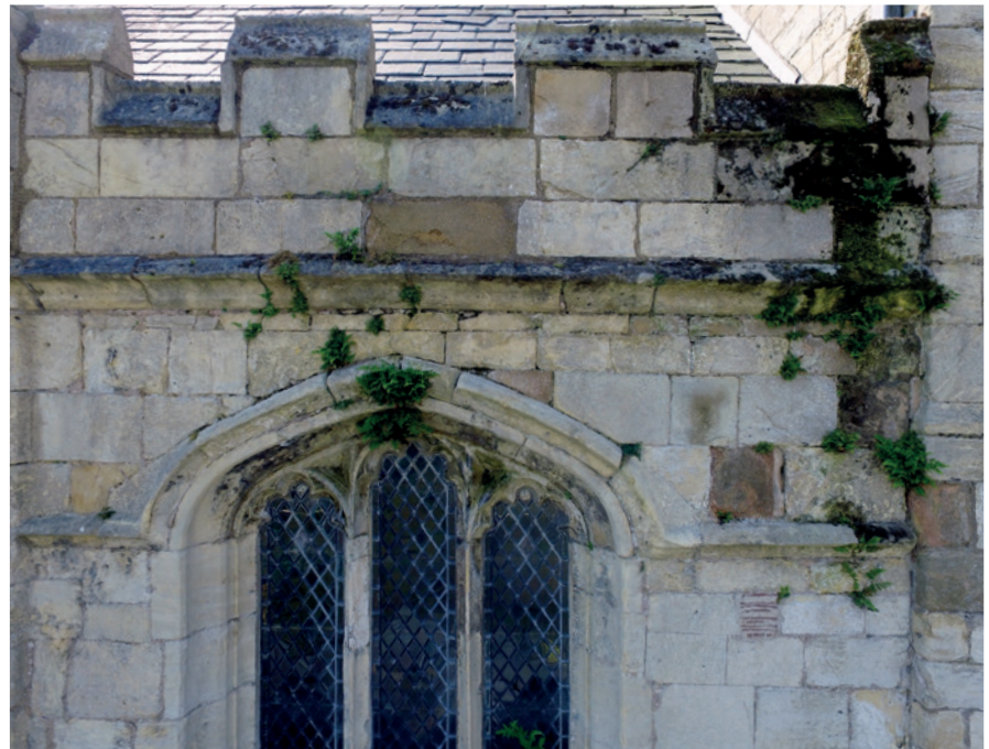
Typical signs of damp caused by an overflowing parapet gutter
