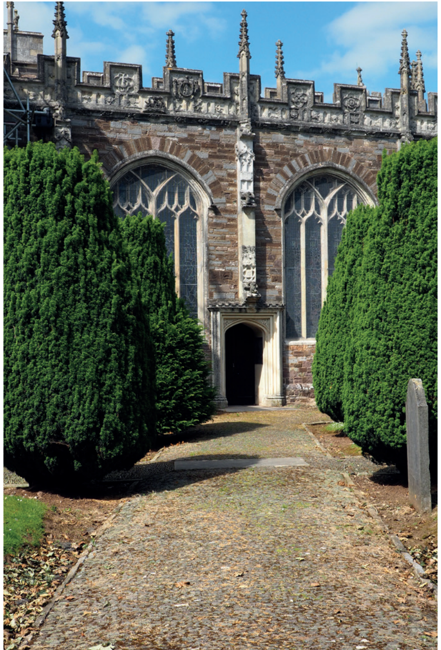
Tightly packed flat-topped cobbles bound by small kerb stones provide a relatively even surface at St Peter's, Tiverton, Devon
