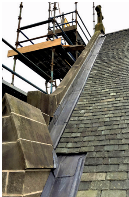
A new 'watergate' with a lead skew flashing and a storm roll to prevent storm water spreading into the sarking
