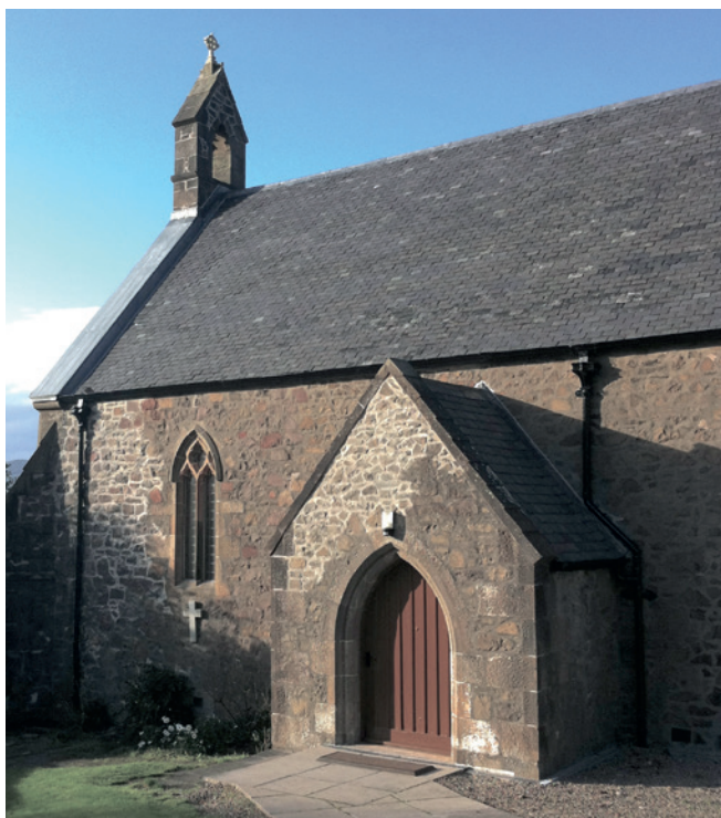
A reslated roof with lead caps to the skews
