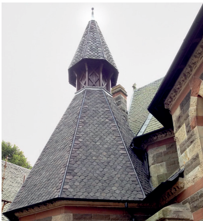
New Welsh slate work on the vestry spire of Trinity, Irvine with code 6 lead roll hip ridges
