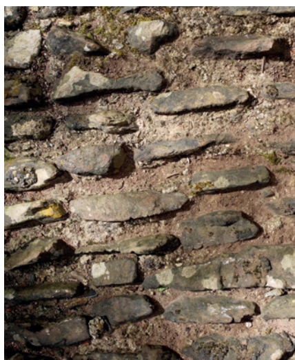
Plants removed from cobble revealing a worn original earth mortar infill
