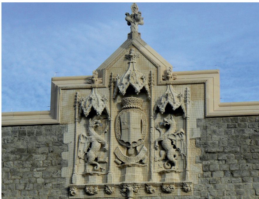
The central crest after consolidation and repair: note the new stone shield, Muscovy hat, copings and foliate corbels with nanolime consolidation and limewash.
