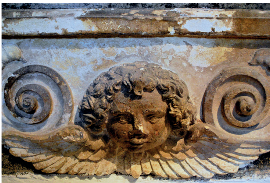
Detail of the lower section of the monument to Sir Edward and Lady Francis at St Leonard's showing salt efflorescence with associated blistering and loss of surface due to raised levels of moisture and salt activity
