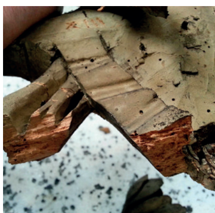
Woodworm damage in carvings of the reredos
