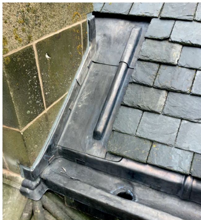
A relined channel gutter with a new watertight detail above
