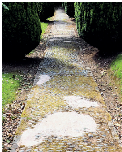
Ugly concrete infill and cement repairs
