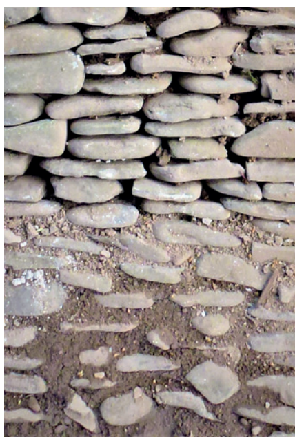
Cobbles partially backfilled with sub-soil, showing the flat-topped form of reclaimed river-worn cobbles
