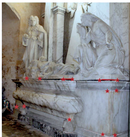
The monument to the Hon Robert Dormer (d1726), Church of the Holy Cross, Quainton, Buckinghamshire, showing the location of the iron fixings and the significant movement through the joints caused by the corroding iron fixings
