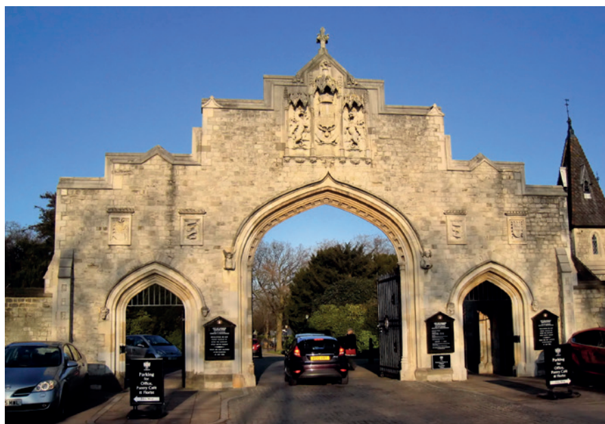
The City of London Cemetery screen before the project: the use of impermeable cement repairs had increased the rate of decay to the point that the stonework had become unsafe. The central shield in particular was perilously close to becoming detached.
