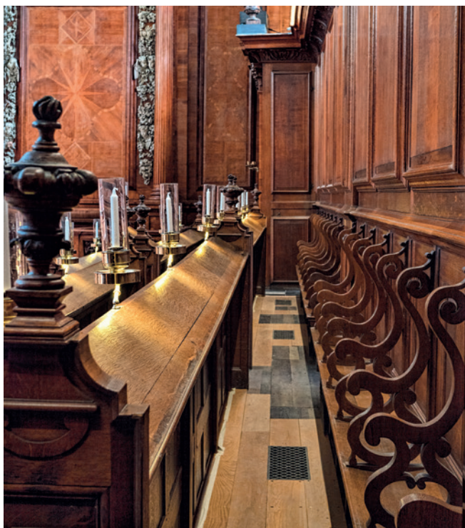
Repairs to the raised floor below the pews, with a mixture of new European oak boards and sections of salvaged originals
