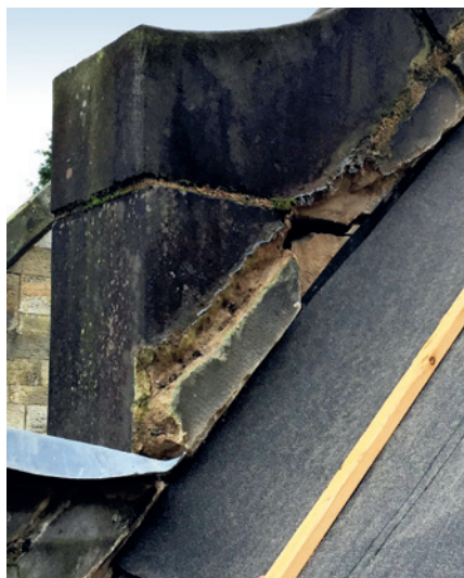
Erosion of skew masonry beneath defective flashings, with flush cope stones above
