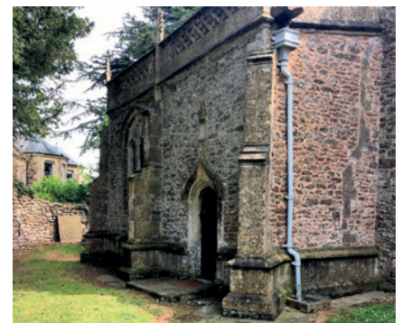
The north and west elevations of the Rodney Chapel showing the lime mortar pointing on the west elevation and the lowered ground level, now re-turfed and sloping away from the base of the stonework
