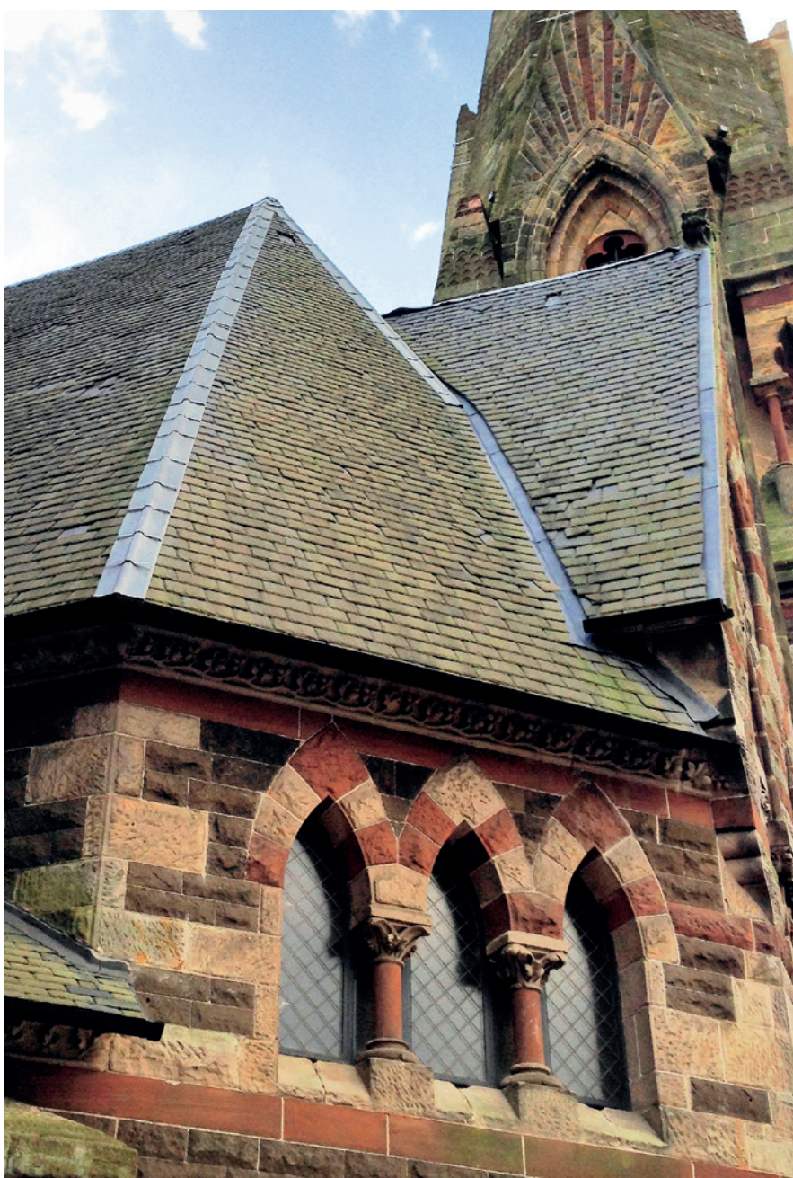
Storm damage to the roof of Trinity Church in Irvine, North Ayrshire due to poor slate fixings and the use of lightweight zinc ridges (All photos: Rebecca Cadie)
