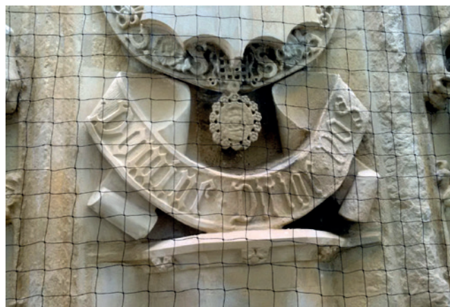
The bottom of the crest completed: note the retained original fine carved medallion and the new shield above it. The friable areas of stone were first consolidated with nanolime, then mortar repaired and limewashed.
