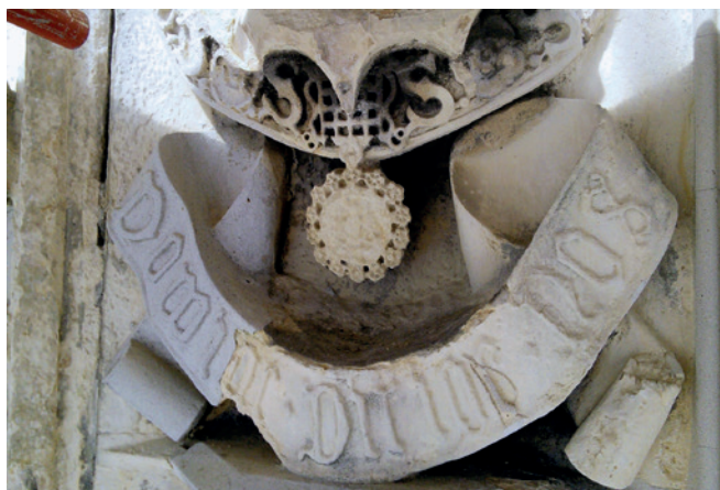
The bottom of the crest before work: note the cementitious repair (left) and adjacent erosion.
