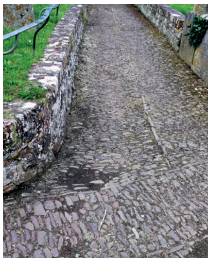
St Swithuns, Sandford, Devon: some areas have sunk and collect water, but otherwise this section is in good repair
