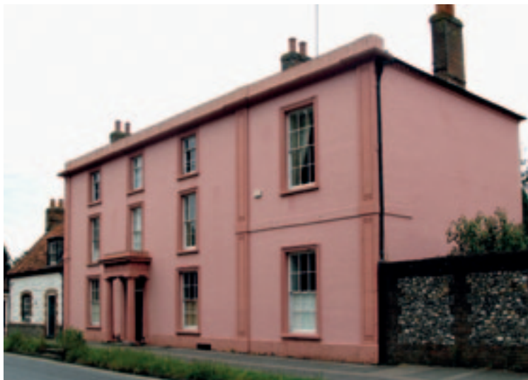
51 High Street, Wallingford: the facade and return elevation of this already painted Grade II listed building were repainted without listed building consent
