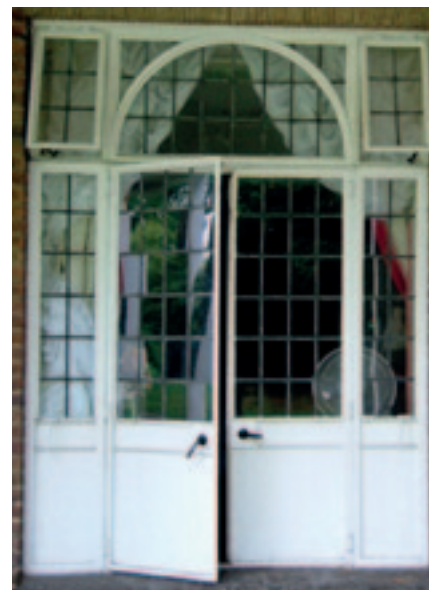
Neo-Georgian glazed metal doors at Elizabeth House
