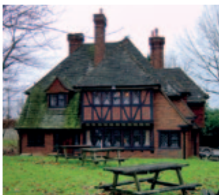
Inter-war steel windows were used to imitate Tudor glazing at The Fox public house, Bix, Oxfordshire, 1936
