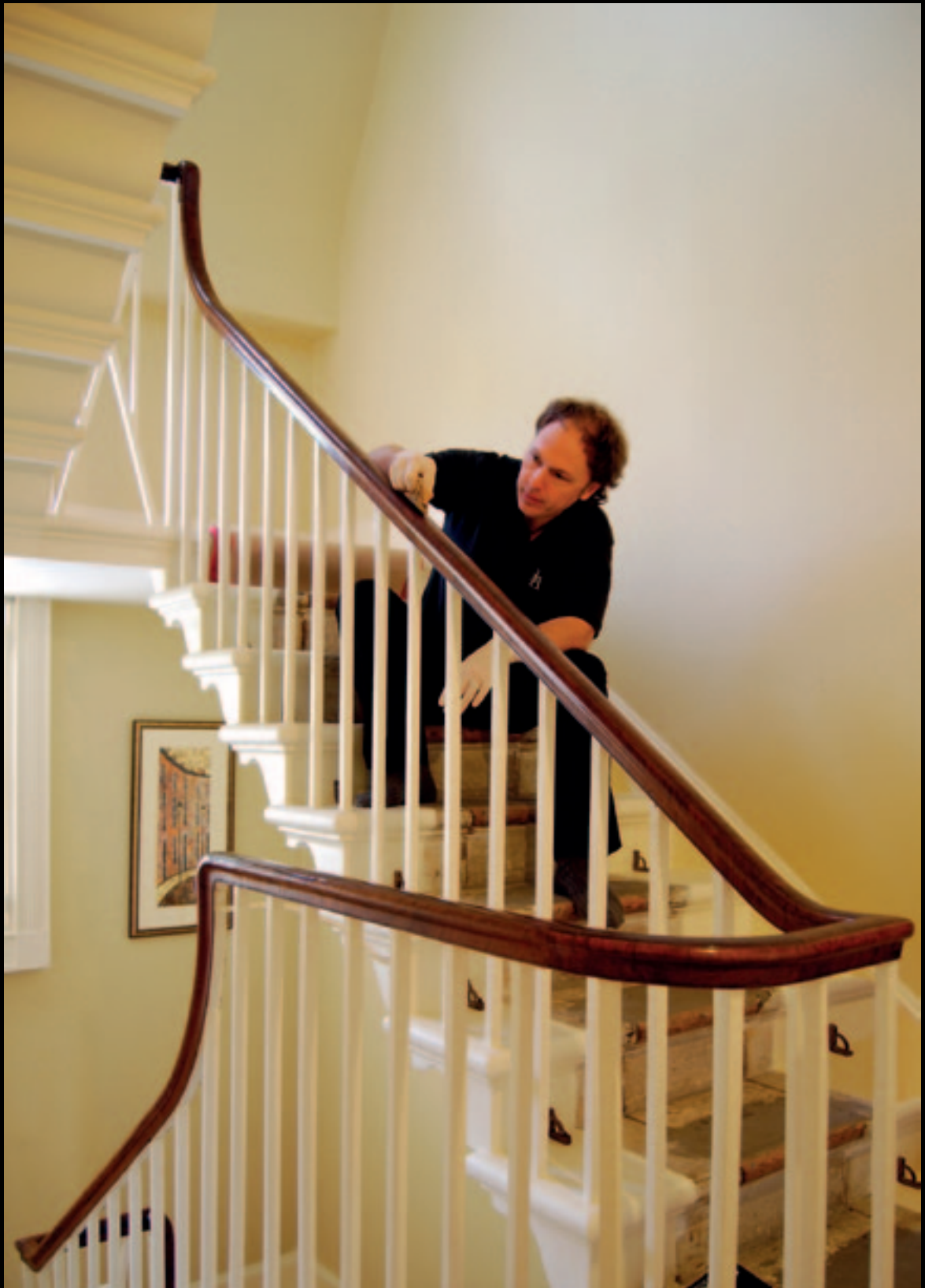
Chris Cole of Banisters of Bath, repairing the cross-banded and French polished handrail of a late 18th century town house in Bath Photo: Jonathan Taylor
