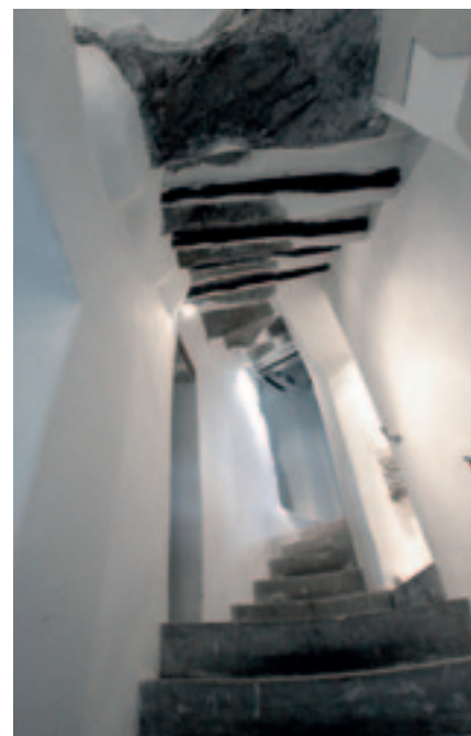
New lime render on the staircase walls
