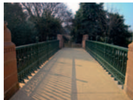
A composite bridge with new resin bound gravel surfacing
