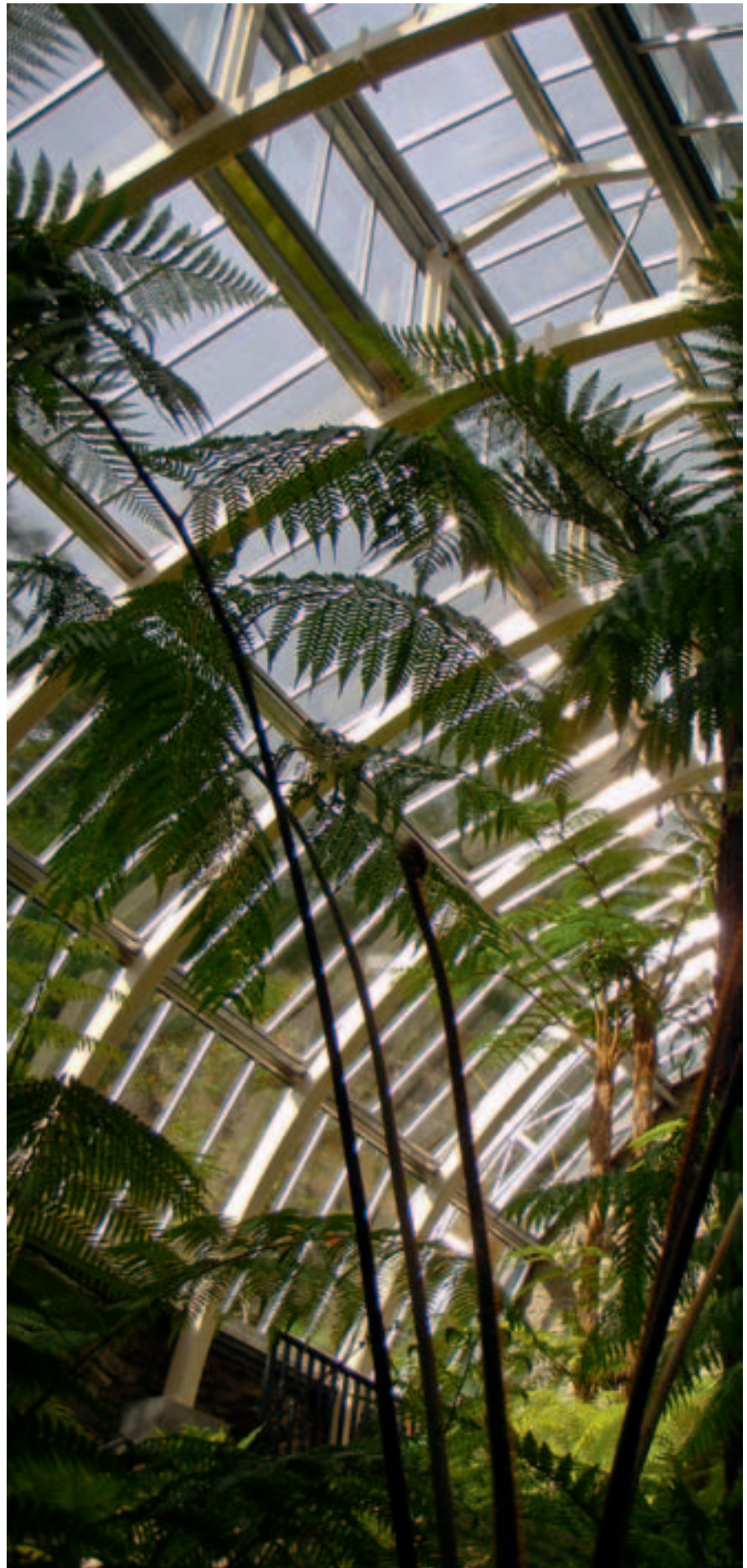
Tree ferns flourishing in the renewed fernery (Photo: MAST Architects)
