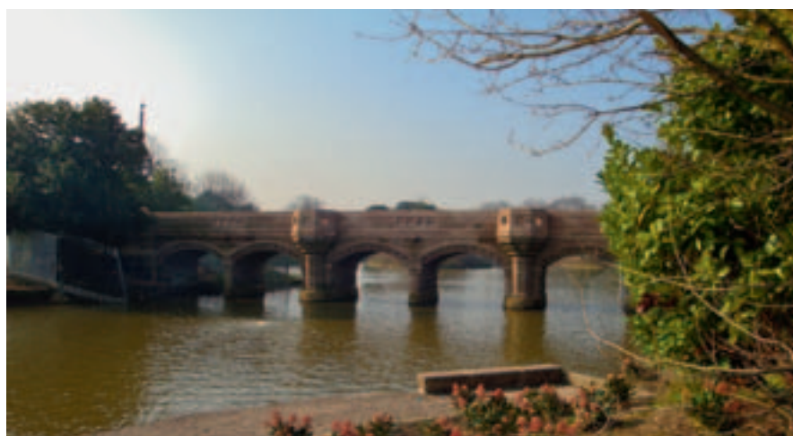
A view of the restored sandstone bridge following reconstruction of the guardings and refuge detail
