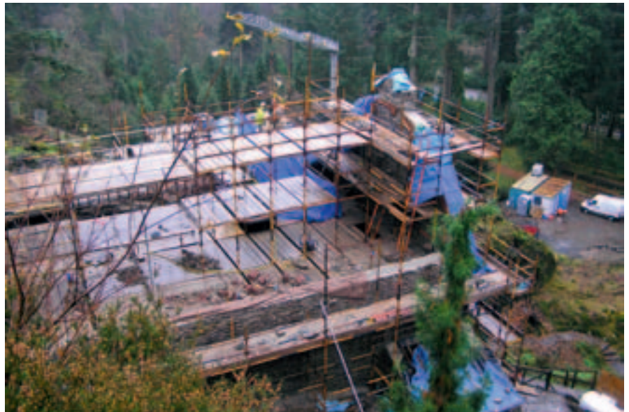
Work in progress (Photo: MAST Architects)
