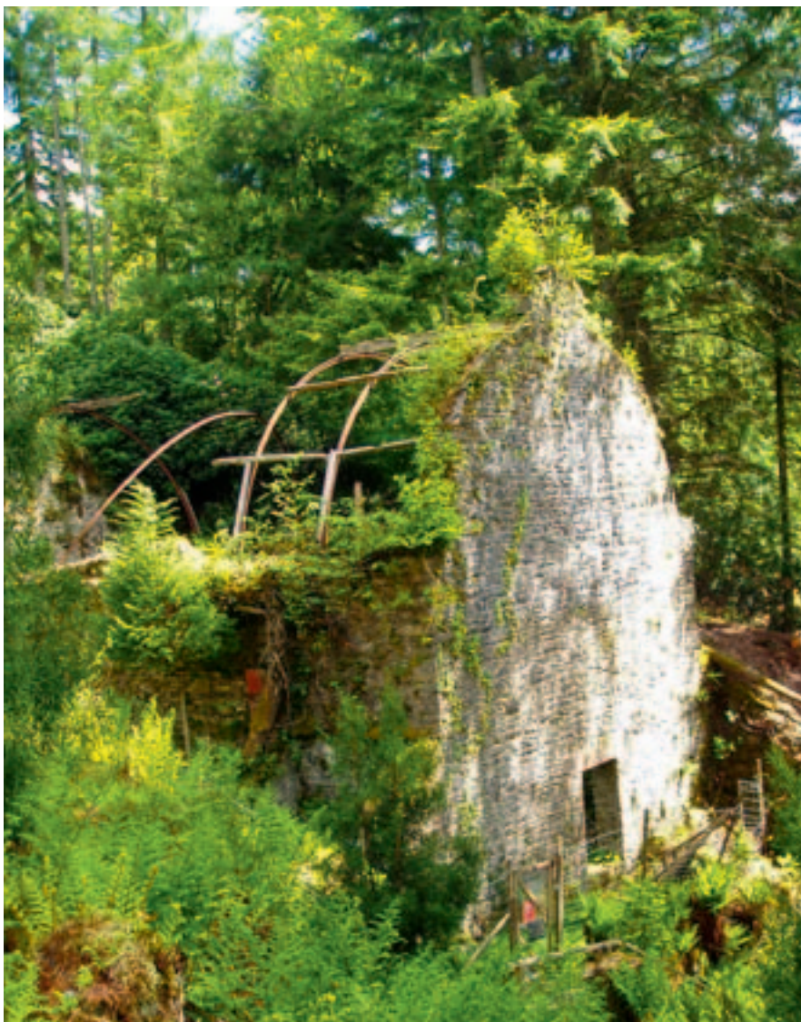
The derelict fernery with its towering south gable (Photo: MAST Architects)
